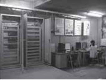
Control room (control panel, PC for control) Photo 2 Test devices
