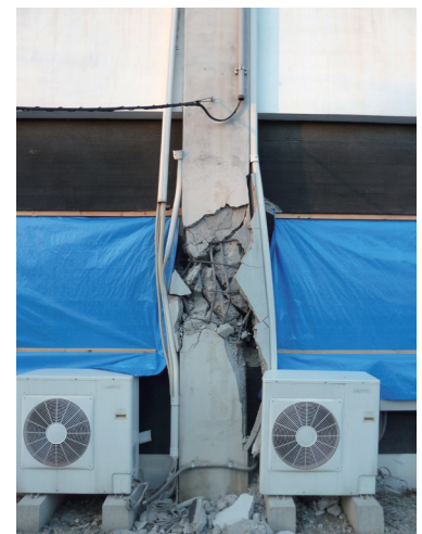
Photo 8: Shear failure
