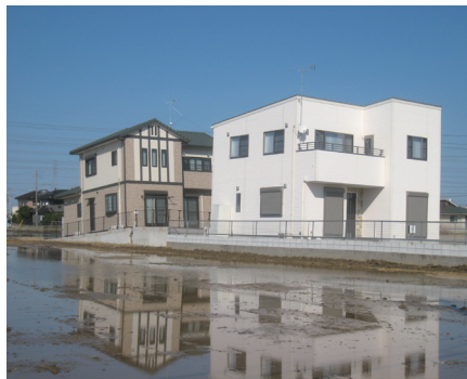
Photo 10: Tilting due to liquefaction
