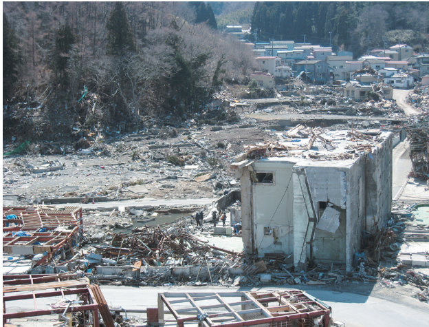
The tsunami swept away all the wooden and low-rise buildings in this coastal area of Onagawa, Miyagi Prefecture, except for a solitary reinforced concrete building.
