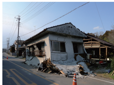
Photo 3: First-floor story collapse
