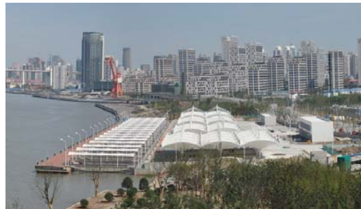
Figure 8: A new visitor ferry service point on the new river bank
