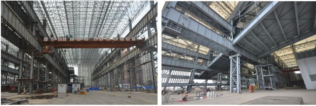
Figure 3 and 4: An assembly workshop for the previous Jiangnan Shipyard were preserved and converted into a museum for shipping industry.
