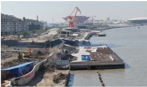
Figure 7: Forming the new river bank along the Pudong strip
