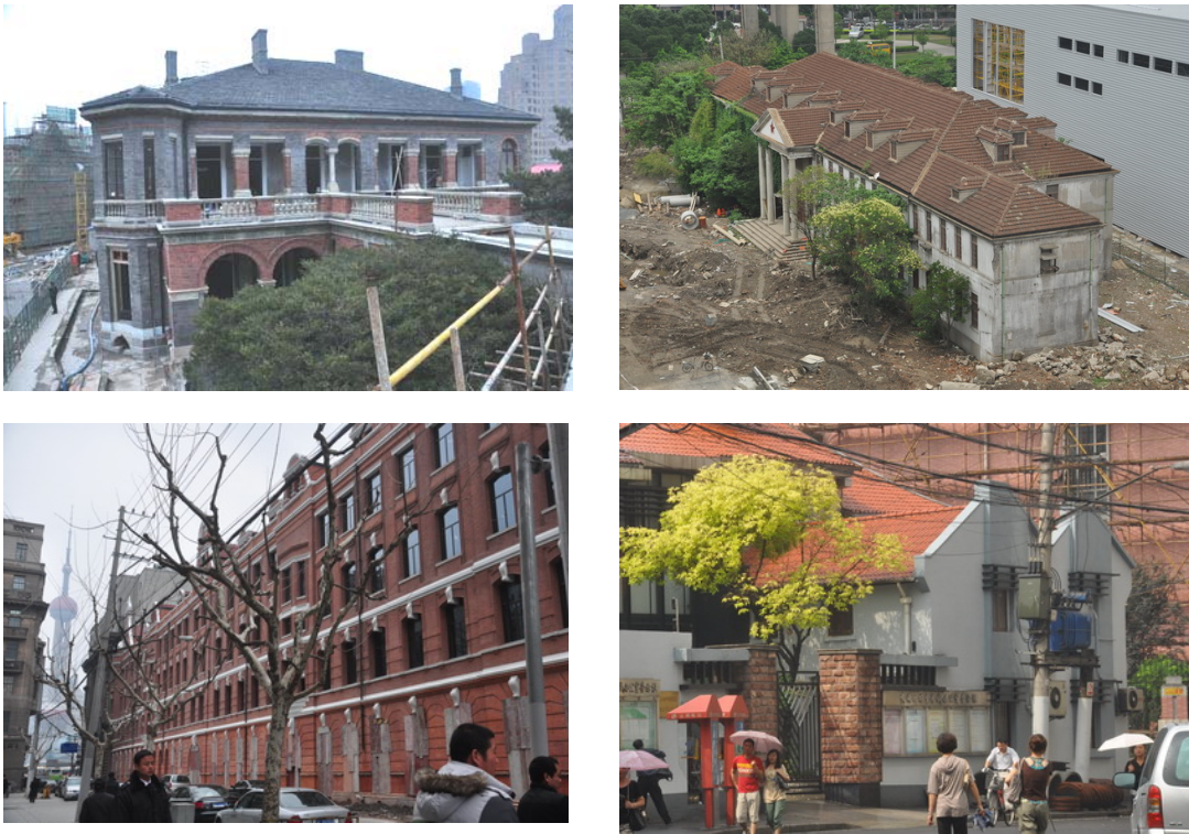
Figure 20: Representing buildings being renovated and converted for other uses
