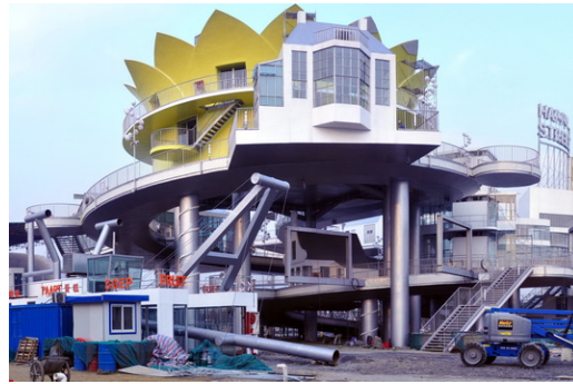
Figure 14: The Holand Pavilion
