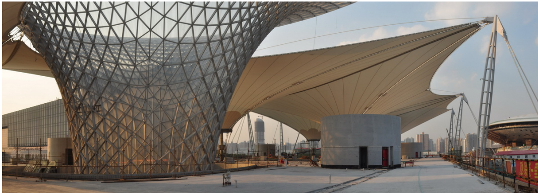
Figure 10: The Expo Boulevard with its eye-catching tent and inverted-cone structures that forms a covered central axis and elevated walkway network that takes visitors to the main pavilions within the Expo principal cores.
