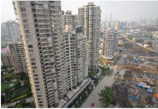
Figure 17: Buildings located just on the touching boundary of the Expo site
